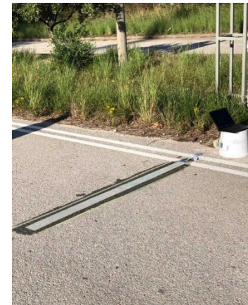
Encapsulated system on the road surface
